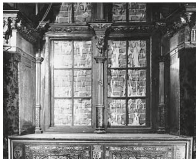
Fig. 5. Window with decorative lights held by lead muntins, the north wall of the Great Council Room. Fragment of a painting by Heinrich Hansen from around the mid-19 th c.
