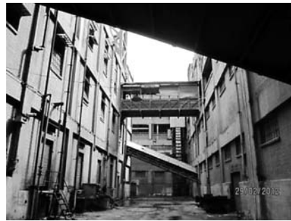
Fig. 22. Current situation inside courtyard of Makbas Elnile showing linking bridges (Source: authors, 2012)
