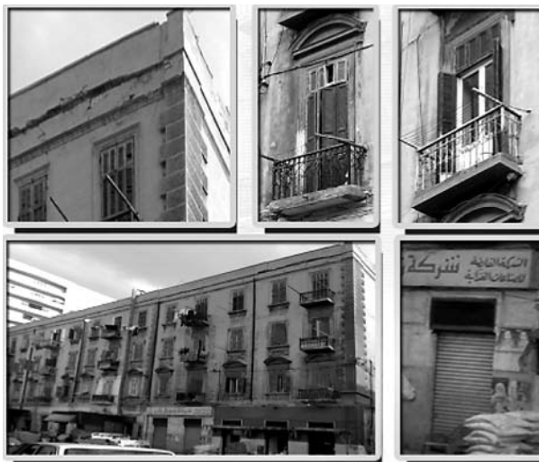
Fig. 12. Photos showing the building façades current condition (Source: the author, 2010)
