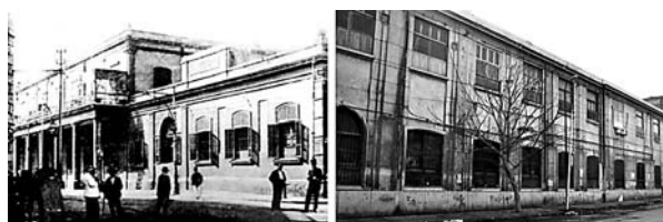
Fig. 4. Left: Old photo of the Bourse of Minet El-Bassal, designed by P. Avoscani 4 , and Right: new photo of the Bourse of Minet El-Bassal (Source: authors, 2012)
