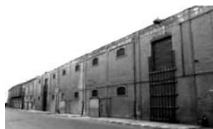
Fig. 15. Warehouse bank Misr, side elevation
