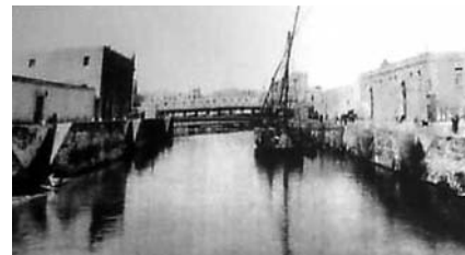
Fig. 6. Map dated 1947 presented to the insurance companies operating in Egypt at that time from the Société Générale de Pressage et de Dépôts. The map shows the ownership of the company [5]; Below: an old picture of the area and Mahmoudiyya Canal [4]
