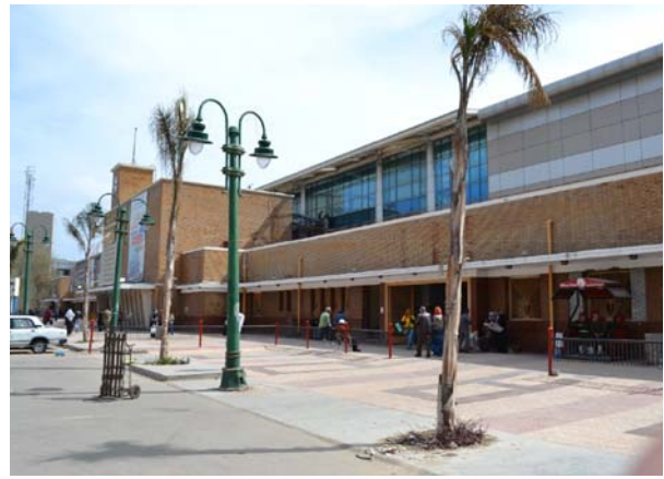
Fig. 6. The new facade with new finishing materials over the old train station building causing aesthetic pollution
