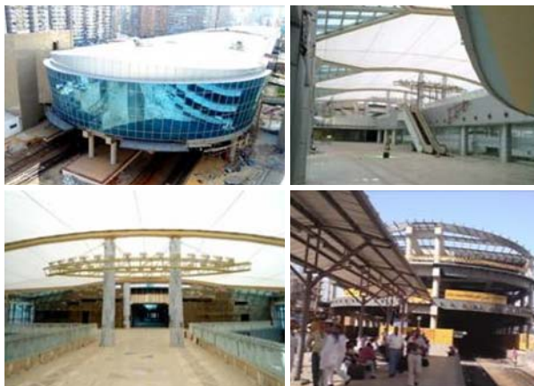
Fig. 5. The new development project of sidi gaber station photos showing the use of modern finishing materials
