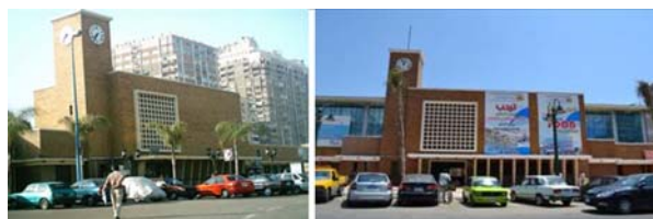
Fig. 3. the old and new facades of Sidi Gaber station
