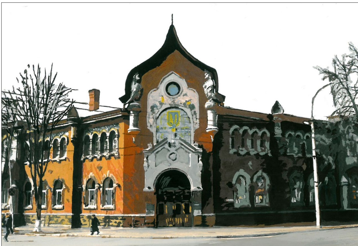
Fig. 3. Present-day view of the Noble and Peasant Bank; the author of the drawing is student V. Otchenko, project supervisor Yu. Ivashko.
