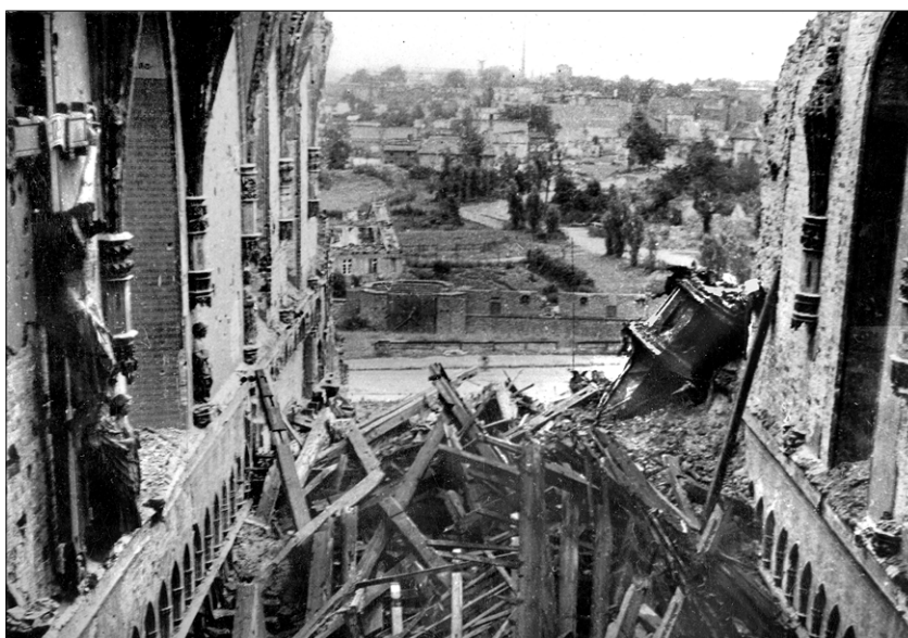
Fig. 2. The interior of the Church, view of the presbytery after war damages, 1945; reprod. by L. Okoński.
