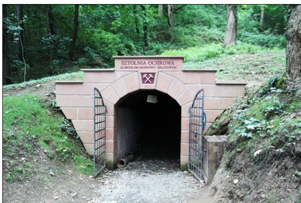
Fig. 6. Gold and arsenic mine in Złoty Stok—contemporary sandstone portal completed when the Ochre Shaft was opened; photo by T. Wieja.
